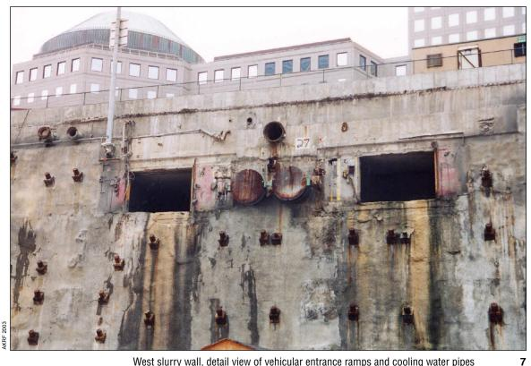
West slurry wall, detail view of vehicular entrance ramps and cooling water pipes
