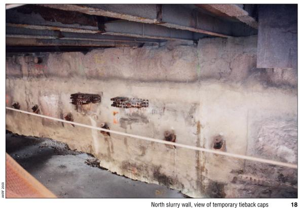
North slurry wall, view of temporary tieback caps
