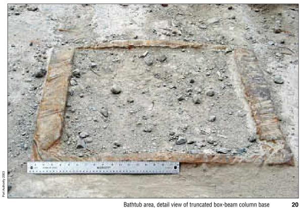
Bathtub area, detail view of truncated box-beam column base
